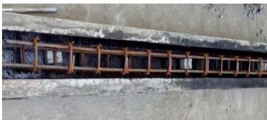
Fig. 1: Mould for beam with reinforcement
