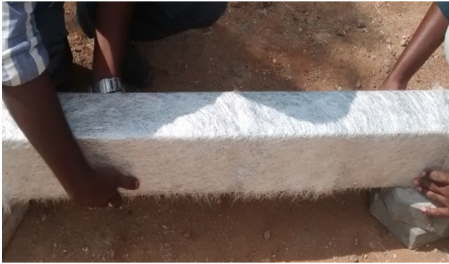
Fig. 4: Wrapping of chopped strand mat
